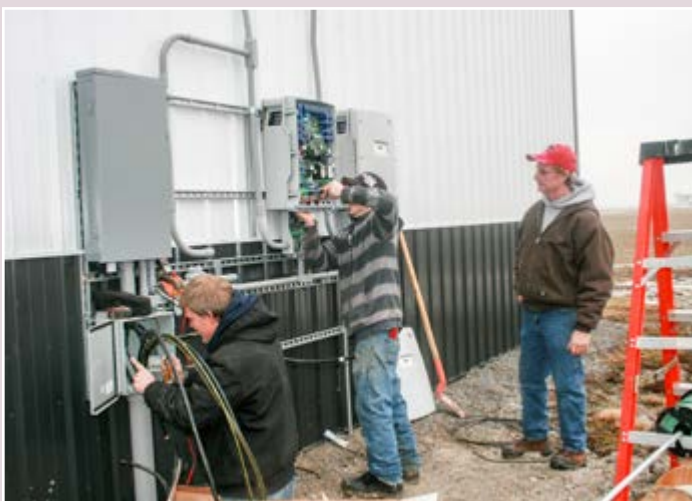
Electricians finish up work on the box
