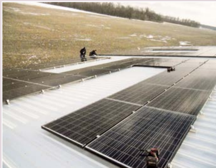
Close-up of solar panels
